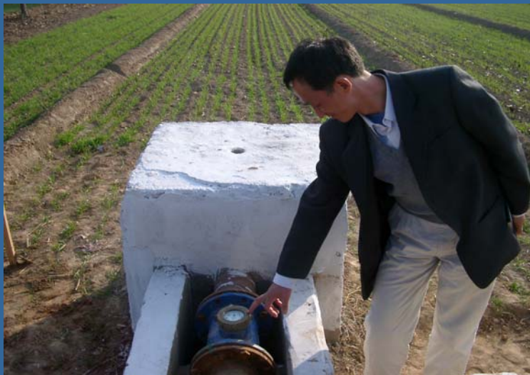
IAIL2 Project Manager checking water meter in buried water distribution pipeline at a WUA in Henan.
