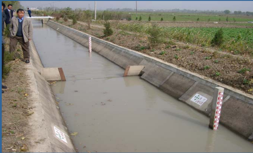
Water measuring facilities at a WUA in Anhui. Water is sold by WSC/water supplier to WUAs by volume. Water measurement is critical, and popular with farmers.
